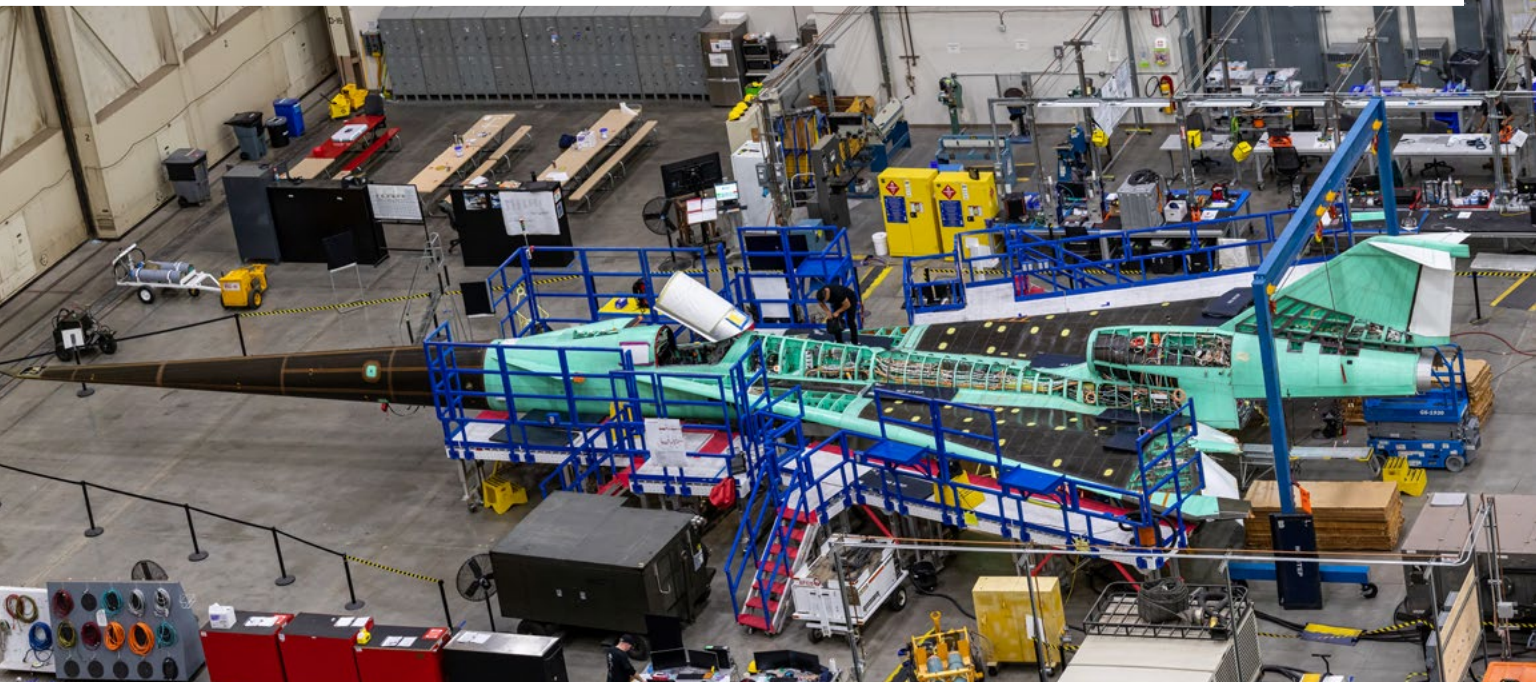
A photo of the X-59 plane being constructed at Lockheed Martin’s “Skunk Works” facility in California
