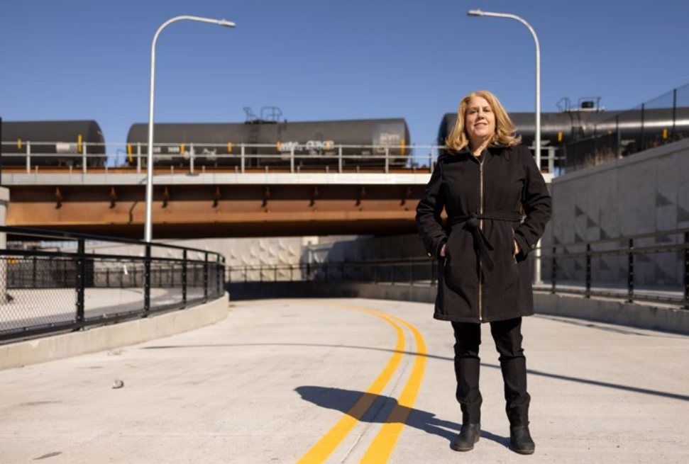
Kris Sorich stands in the middle of a newly built road in The 78 development on Chicago's near South Side. Sorich has played a key role in the development of landscape architecture components of the project, including the pattern of the retaining wall [as shown on the right] and the black gates on the side of the road [left]. PHOTO: TIM KLEIN
